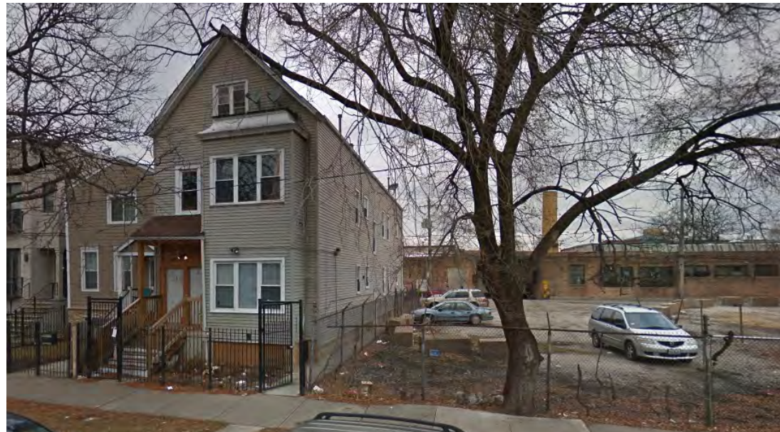
Cortland Street - Adjacent Building
